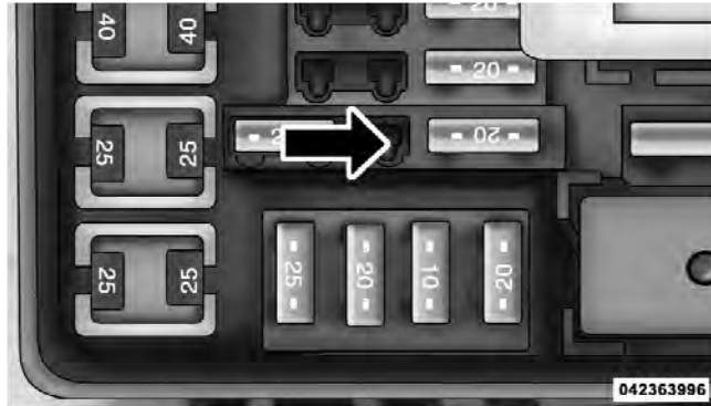
Power Outlet Right Rear Quarter Panel Fuse
