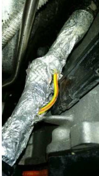
Fig. 4 TCM Wiring Harness Damage
